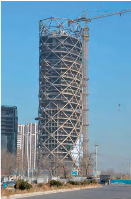
Fig. 6: The Poly Diamond Lantern employs a shallow angle to the diagrid.
