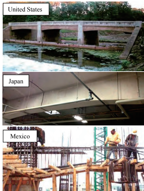
Fig. 1: RC structures with haunched beams
