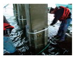
In 2006 DAS anodes installed in concrete jackets for 764 reinforced concrete piers supporting Robert Moses Causes, Long Island, New York, USA. Polarization is well above 100mV and the projected service life is more than the design service life of 35 years.
