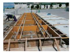
DAS anodes were installed in the precast slabs to prevent corrosion from initiating in aggressive environment, White Beach Piers, US Naval Base, Okinawa, Japan.
