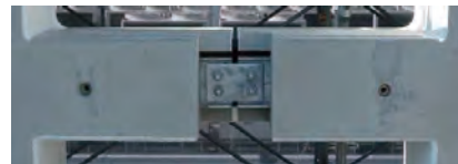
Fig.6 joint (girder-girder)
